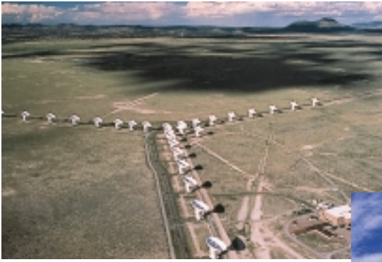
Figure 5.37A The Very Large Array is a Y-shaped array of 27 identical, 25 m dishes on railroad tracks. Electric cables connect the dishes. Each of the three sections of the Y is about 20 km long. The VLA has a resolution so fine that the centimetre marks on a ruler could be seen 5 km away — if the ruler were broadcasting radio waves!
