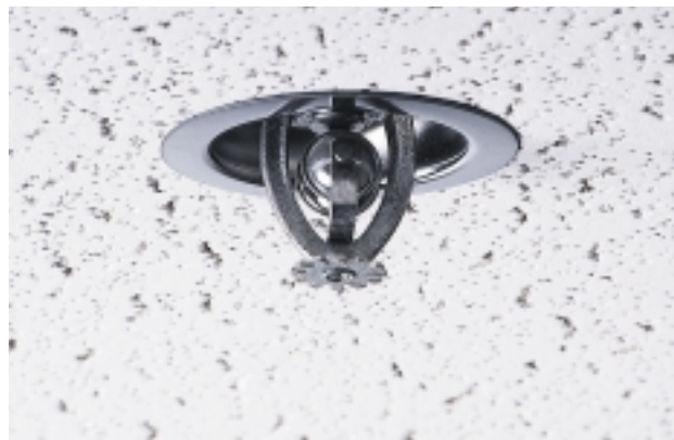
The trigger in this overhead sprinkler is made from bismuth.
