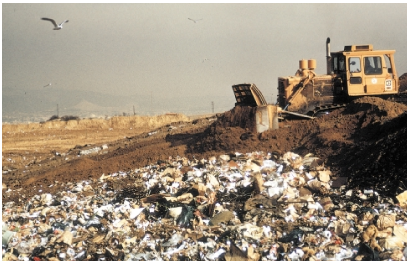
Figure 3.26 Bulldozers pack down trash at a municipal landfill site.
