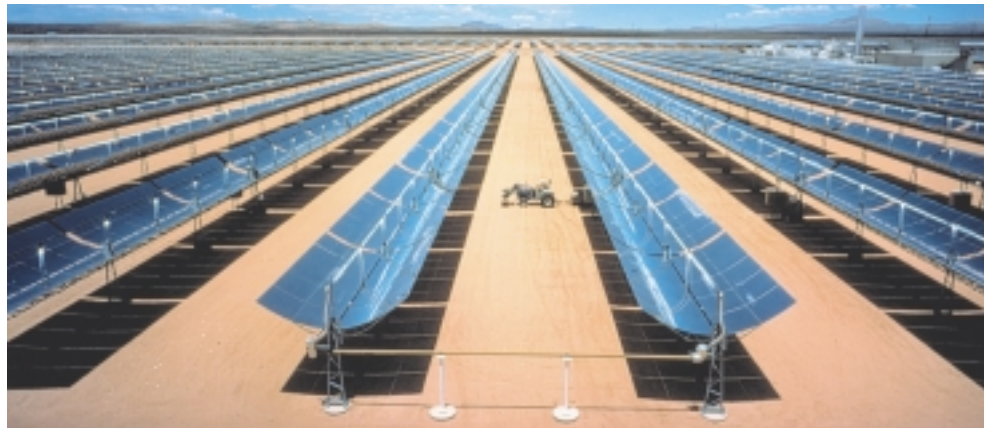
Figure 4.56 Reflective mirrors in the California solar farm are precisely curved to concentrate solar energy on oil-carrying pipes.
