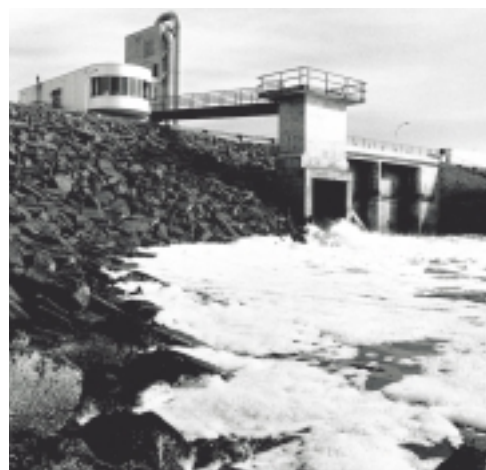
Figure 4.57 The tidal powerhouse is quite similar to a hydro-electric generating station in a dam. As the water that has been trapped in the basin flows out, the water pressure turns turbine blades that turn an electric generator.
