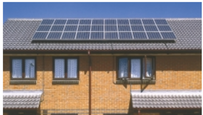
Figure 4.28 Light hitting an individual photovoltaic cell transfers energy to electrons, starting a current through the load. A rooftop solar array can power a house.
